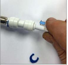
• Push the hose firmly into the white collet of the push-fit fitting until it stops.
